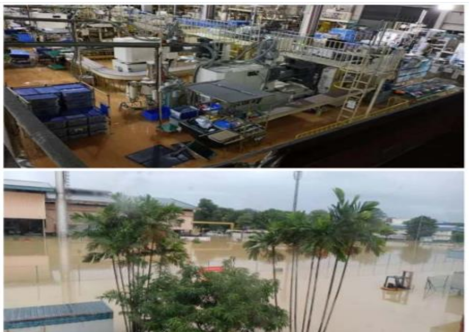
Figure 4: PMM's SA2 plant in Shah Alam was inundated by floodwaters
