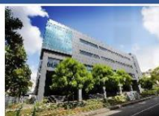
8 Commonwealth Lane ("8CL")
