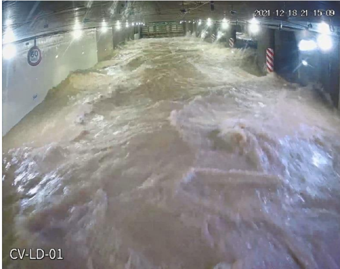
Figure 27: SMART Tunnel at full activation
