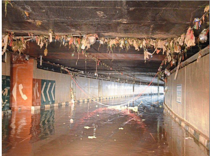
Figure 28: SMART Tunnel water diversion in progress
