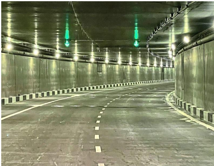
Figure 29: SMART Tunnel clean up post-water diversion
